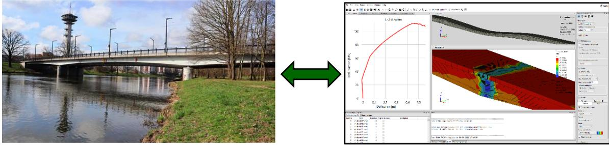
**Fig. 1.** Digital Twin involves active data exchange between the real structure with monitoring sensors (left) and virtual twin, i.e. its numerical model (right).
