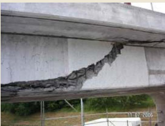
The loaded span has been meshed with volume elements, for the other span, a coarser mesh of shell elements has been used. The most important reinforcement has been modelled with discrete bars, the rest by smeared reinforcement. In the Load-Displacement graph you can see how close are the analysis results to the measured response. You can also compare the calculated crack pattern with the final shear crack.
