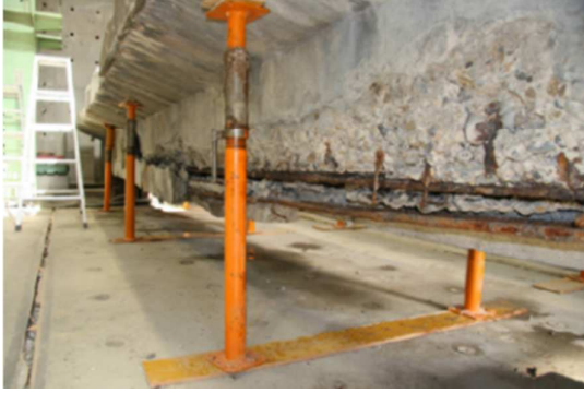
Figure 3: The validation beam from the Nougawa bridge [15]
