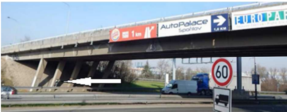
Figure 8: View of bridge with the analyzed strut
