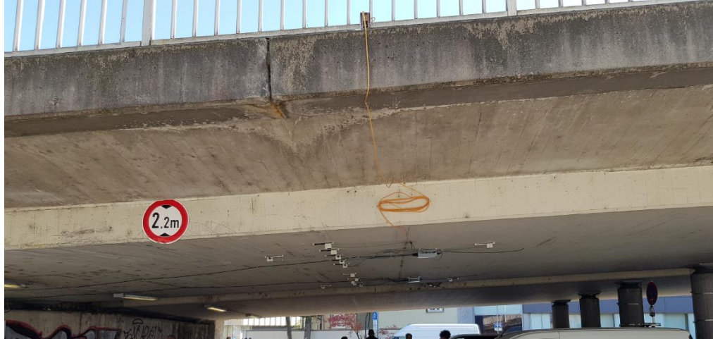
Figure 7. Digital Twin monitoring application at Vogelsang bridge in Germany.
