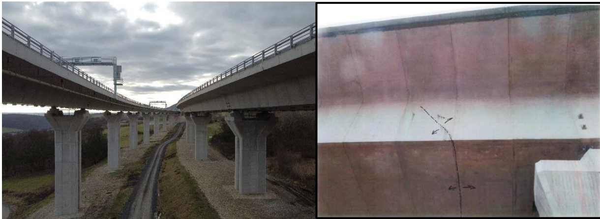
Figure 5. A view of the investigated viaduct.
