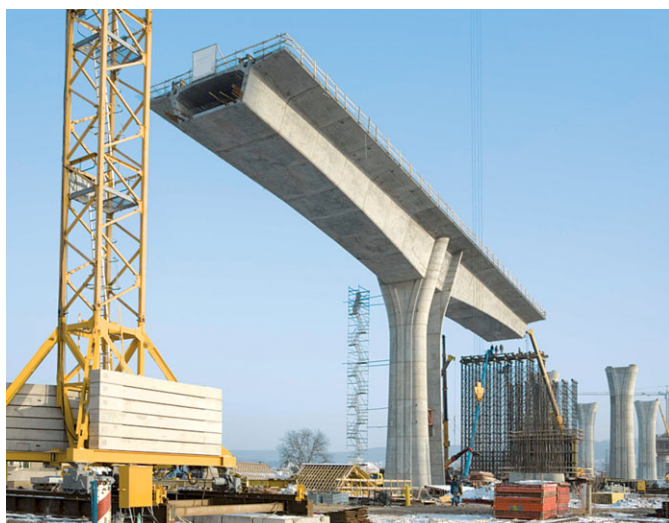
Fig. 11. Bridge under construction, built using the balanced cantilever method
