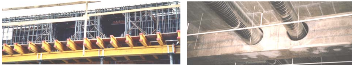
Fig. 12 Reinforcement detailing (left). Finished girder with opening (right).
