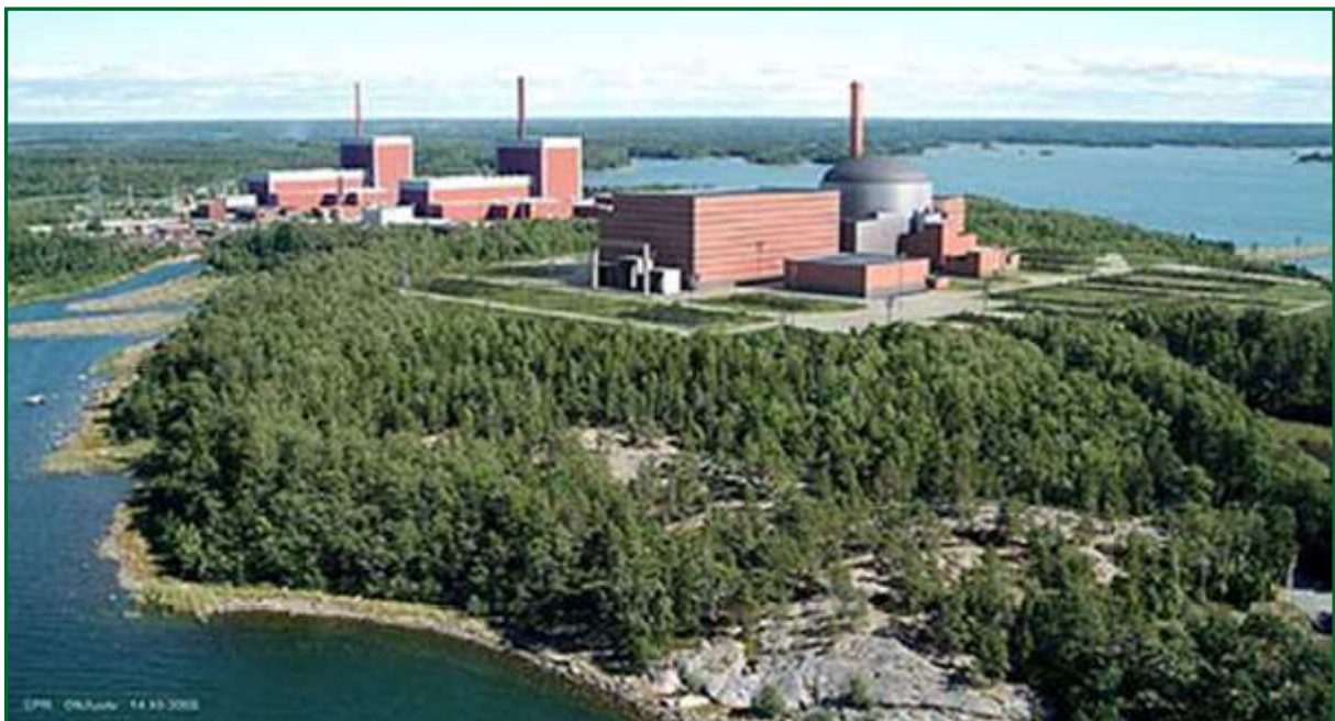
Figure 1 The newly constructed nuclear power plant Olkiluoto 3 in Finland was also analyzed with ATENA.
