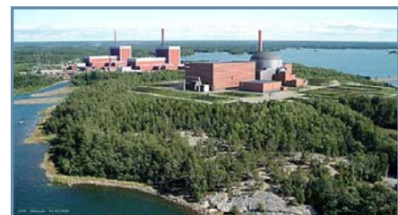
Olkiluoto 3 nuclear power plant in Finland
